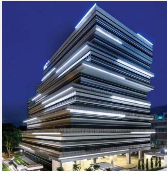
100PP OFFICE BUILDING
