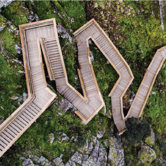
TRIMETRICA - PAIVA WALKWAYS
